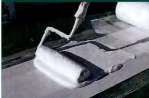
STEP 4: Apply liquid adhesive
