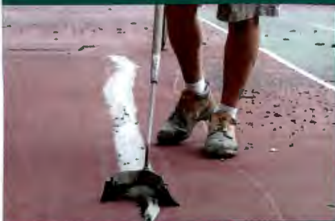
STEP 1: Fill cracks up to 4 inches wide
