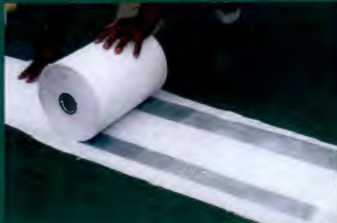
STEP 5: Install narrow ARMOR ® fabric
